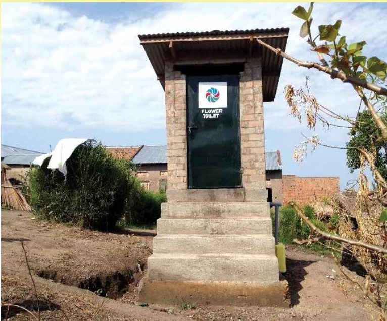
Photo 21: One of the eco-san constructed using ISSBs made by the project in Nyakeera
