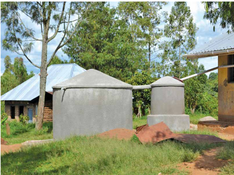
Photo 16: A newly completed 10 cubic metre tank at Kabahango Primary School
