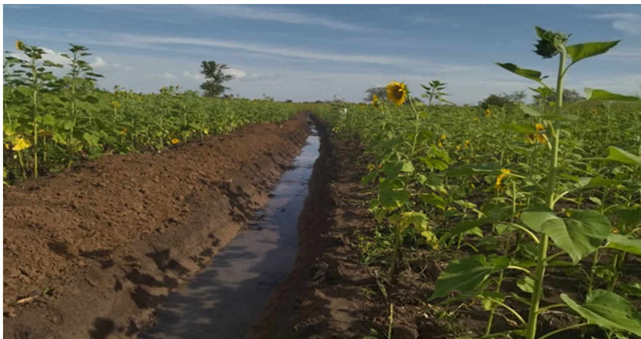
Newly constructed flood control trench in Kamonojwii, Agago District.
